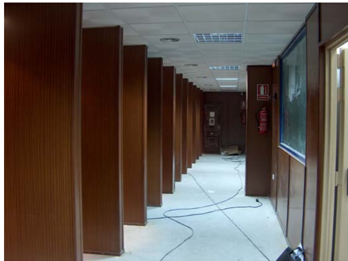
Shooting booths and control room to the right.
